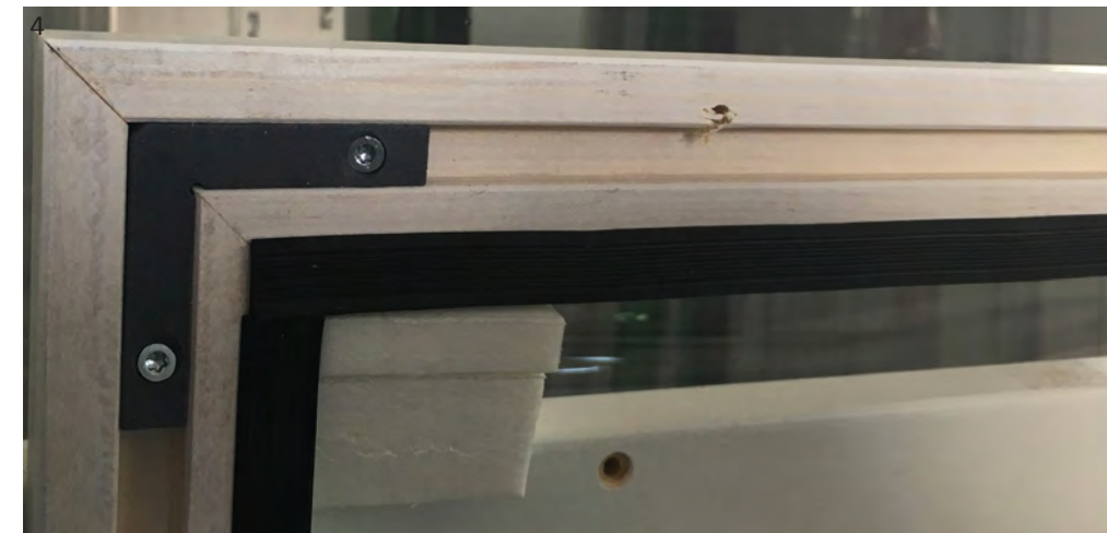
4 Corner bracket fixed with two screws in window assembly
