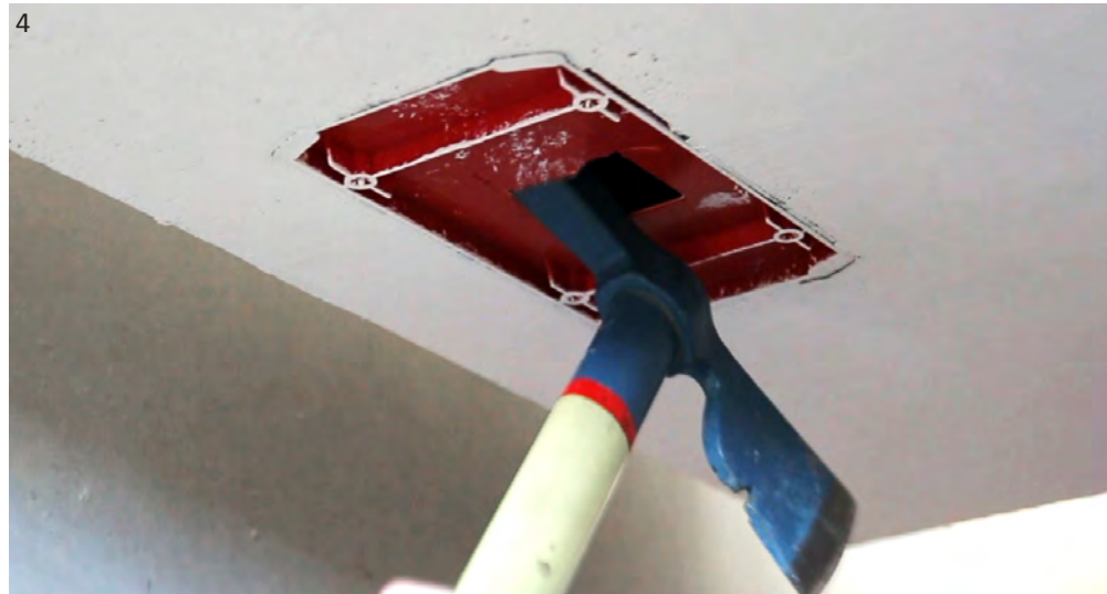
4 Removing the protective cover of the mounting plate
