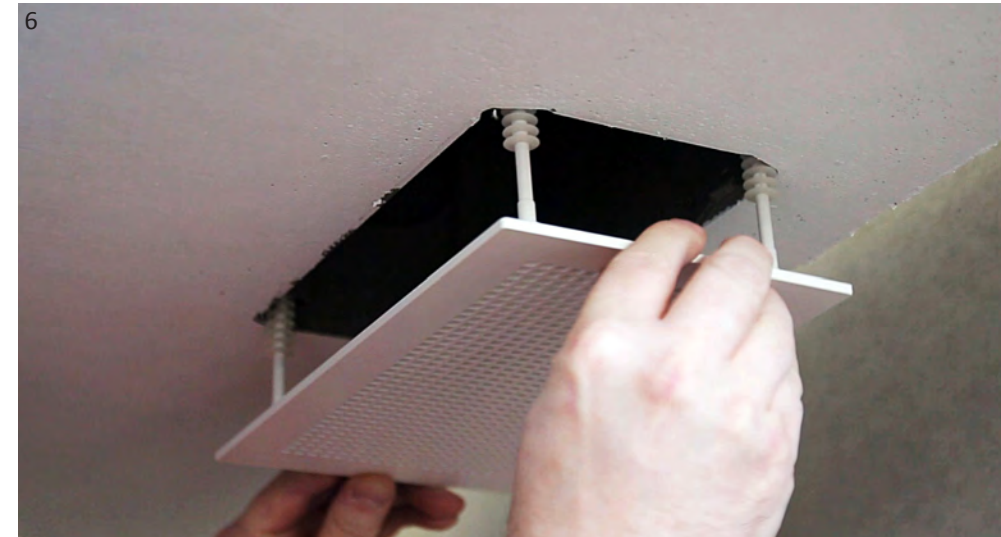
6 Attaching and positioning the ventilation lattice
